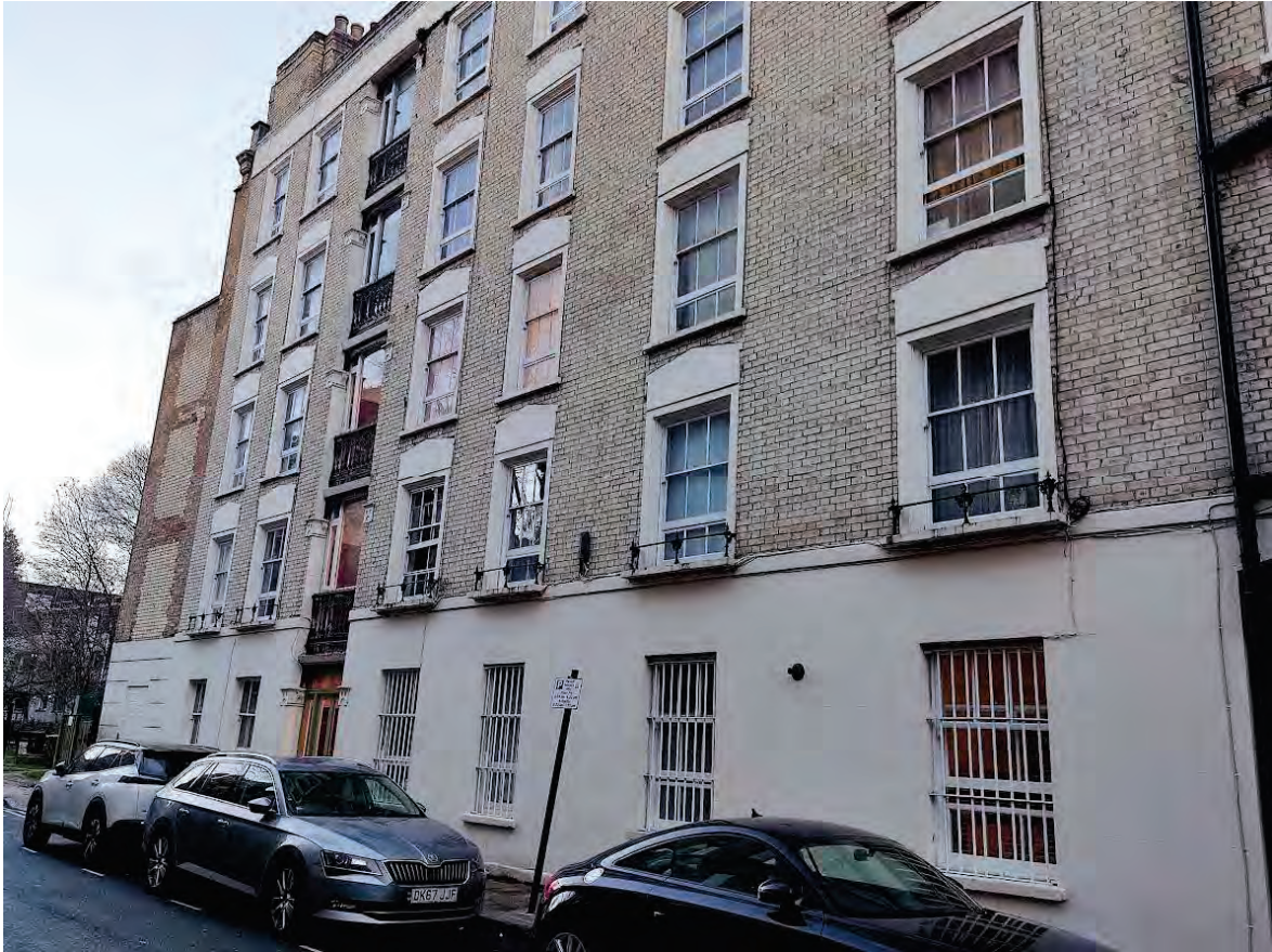
Figure 3: Victoria Chambers, Mark Street façade shown
